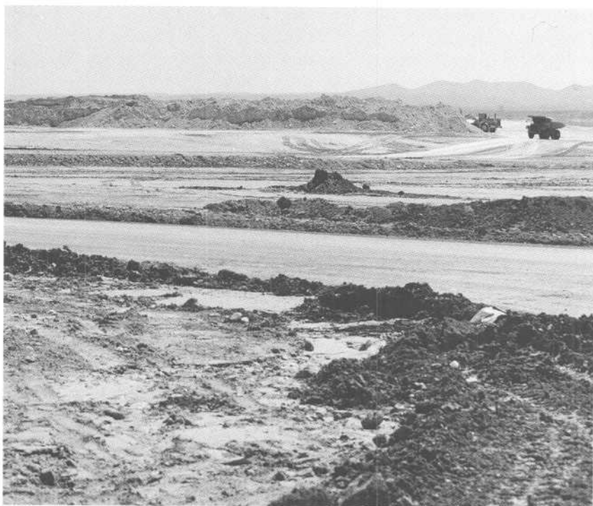
Excavation of Glide Path Hill at Ramon
